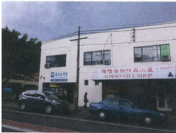
PICTURE 1 – VIEW NORTH WEST ON CAMPSIE ST SHOWING LATER TWENTIETH CENTURY EXTENSIONS TO 140-142 BEAMISH STREET
