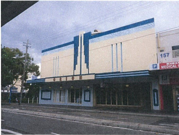
PICTURE 11 – THE ORION CENTRE
