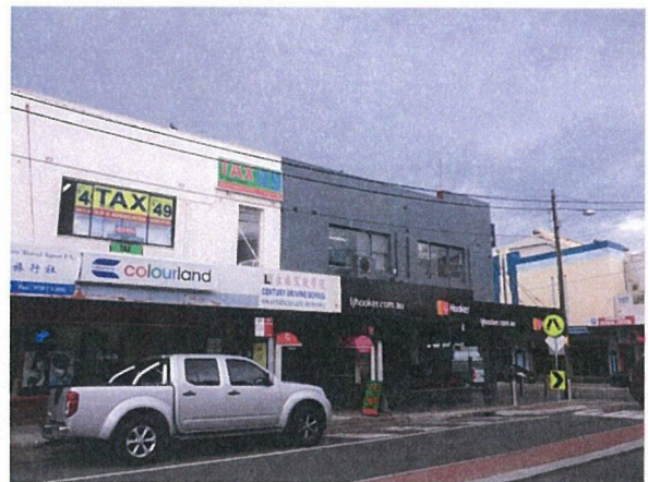
PICTURE 2 – VIEW NORTH EAST ON CAMPSIE ST (TOWARDS BEAMISH STREET)
